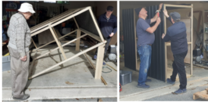
Carparking Shed Construction
