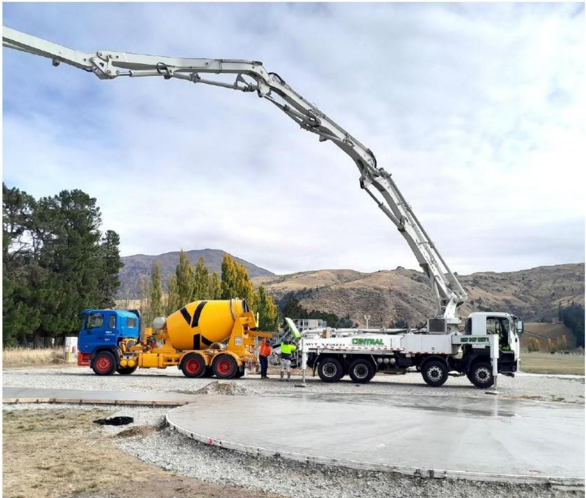
Concrete is being loaded into the hopper then pumped onto the ambulance pad on the helipad site
