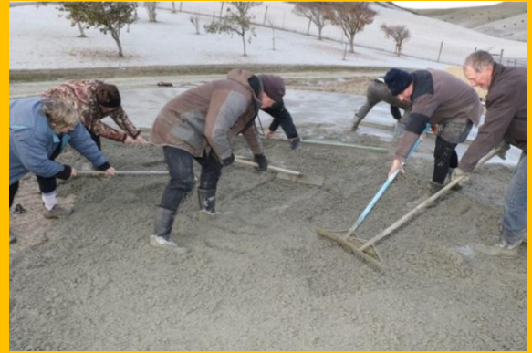
Lawrence Lions screening the concrete for the new heli pad.
